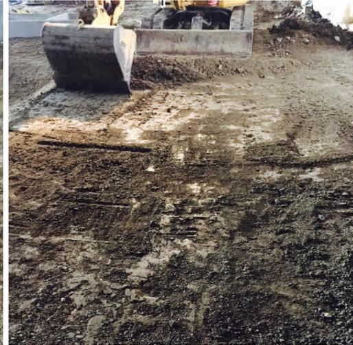
Condition of existing subgrade during winter excavation Partial removal of subgrade for Tough Cell® installation
