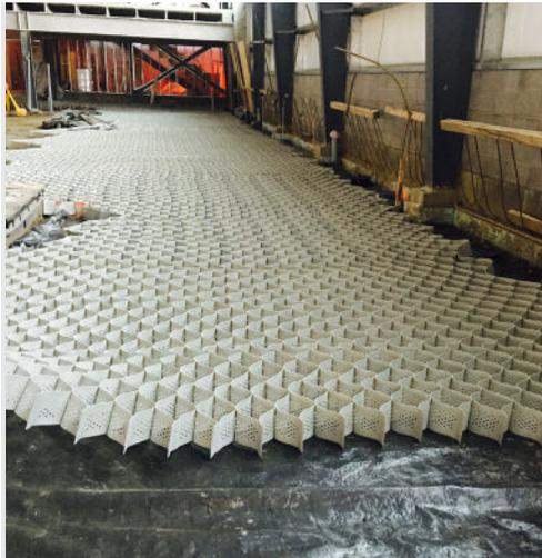
Tough Cell® installed over woven geotextile
