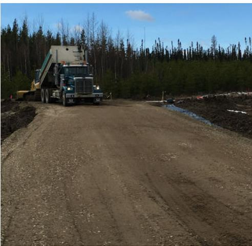
Infilled section supports heavy load during construction
