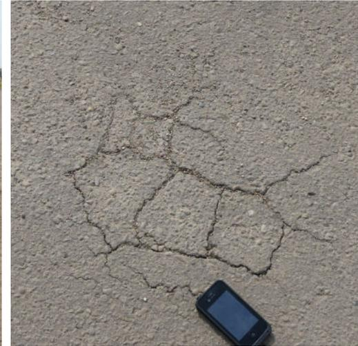
Fatigue cracking in road surface before construction
