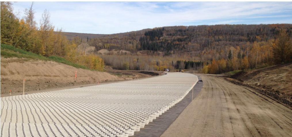
Tough Cell® road constructed in parallel to allow continuous traffic flow during installation
