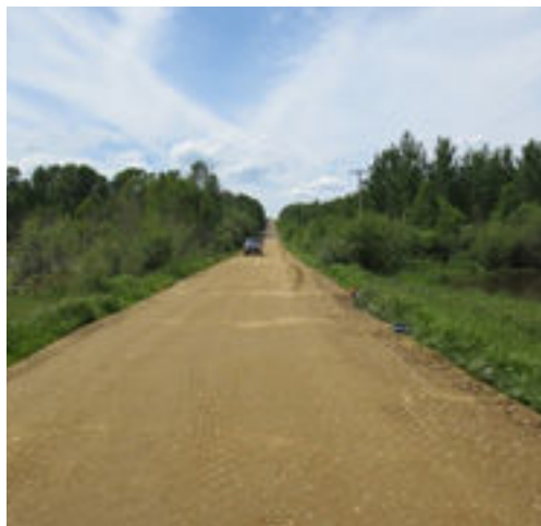
Completed road, June 2013
