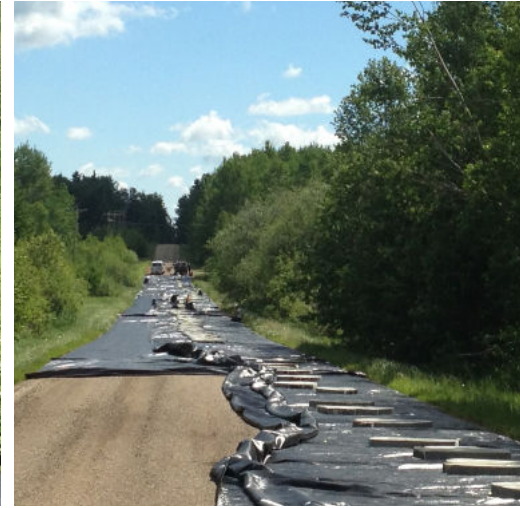
Installation of geotextile layer
