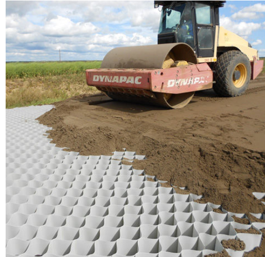
Sand infill and compaction
