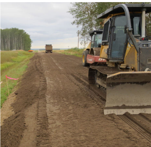
Top course compaction and finishing
