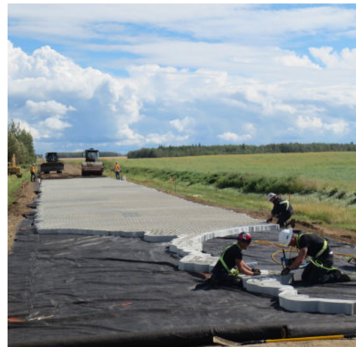
Installation of geotextile and Tough Cell sections.
