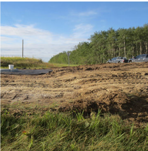
Pre-grading to accommodate elevation change and guard web edges from snagging
