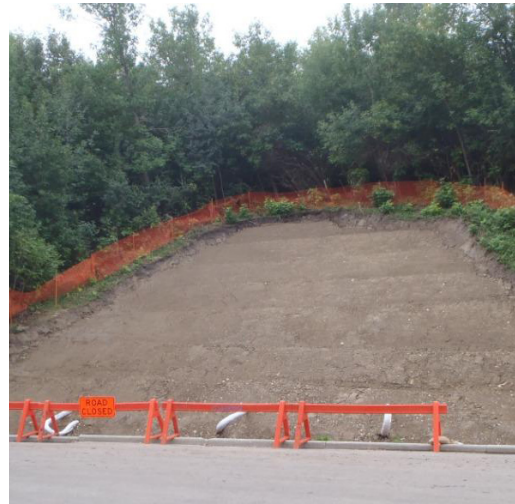
Graded and terraced slope
