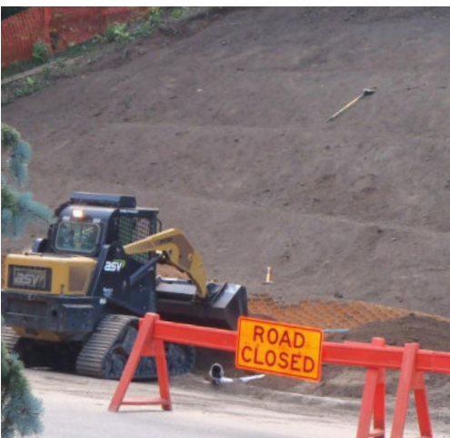
Infilling of Tough Cell ® geocells
