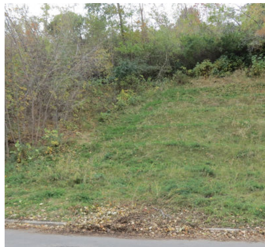
Remediated slope 1 year after install
