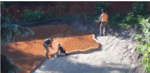
(top) Anchoring of Tough Cell ® to ground (bottom) Installation in progress
