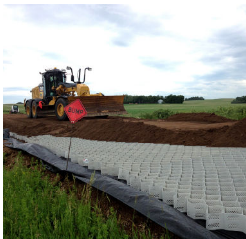
Infilling of Tough Cell® geocells
