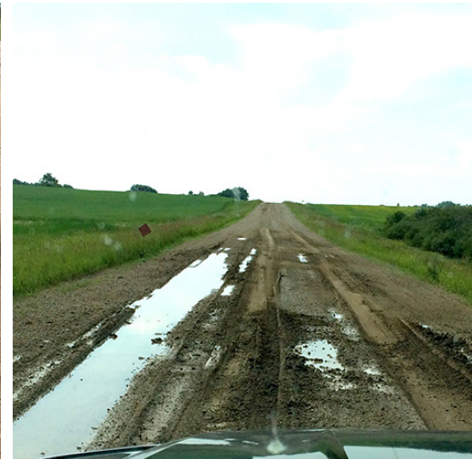
Roadway conditions after heavy rain
