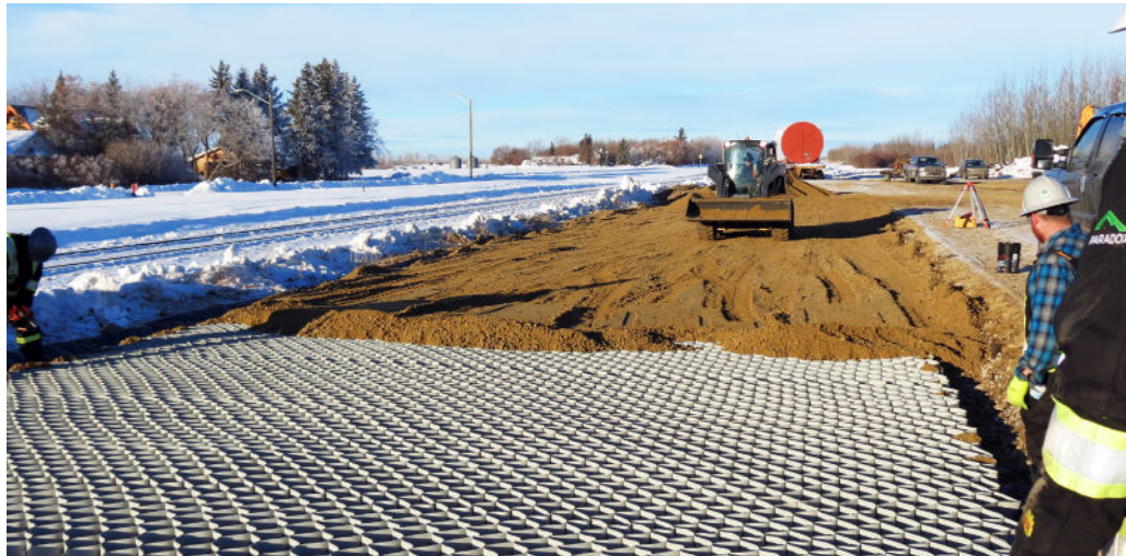
Installation and infilling of Tough Cell®
