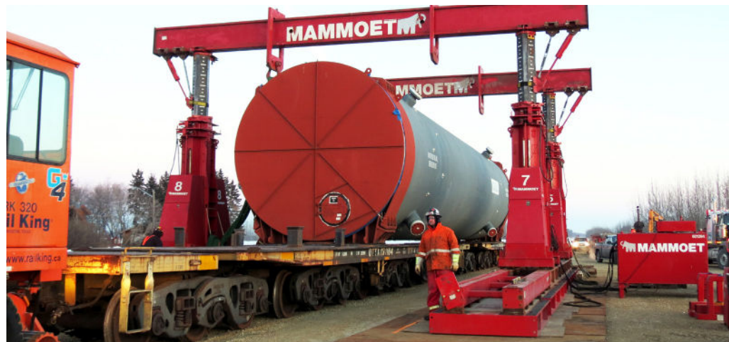
Crane installed and in operation.
