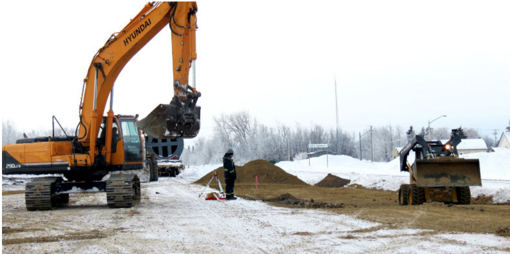
Preparation of base during winter conditions.
