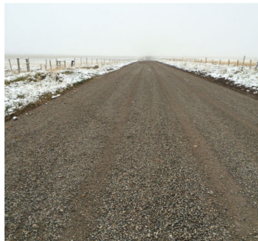
Completed, rehabilitated road surface after install
