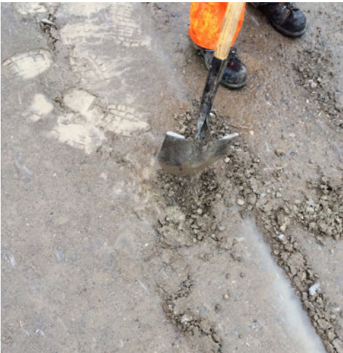
Existing road conditions prior to rehabilitation
