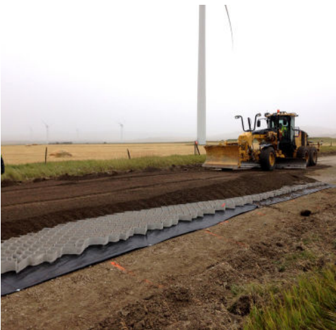
Infilling of Tough Cell® geocells
