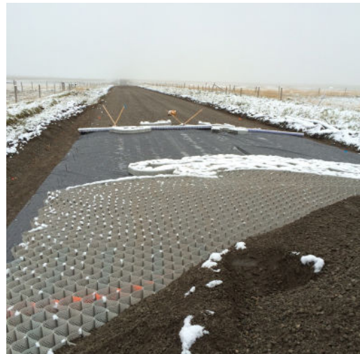
Woven geotextile and Tough Cell® geocells installed in winter conditions
