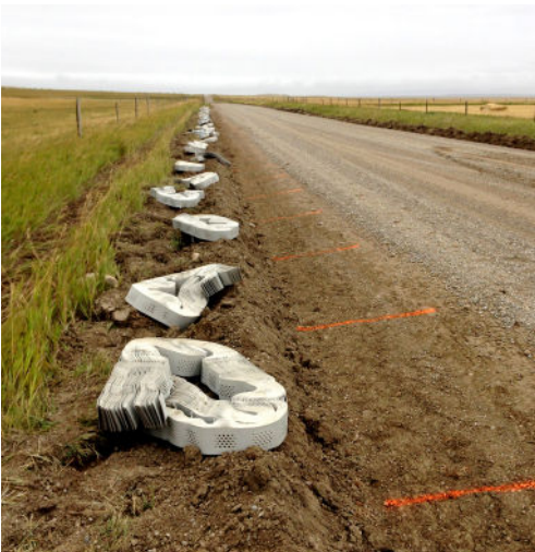
Tough Cell® geocells placed for installation
