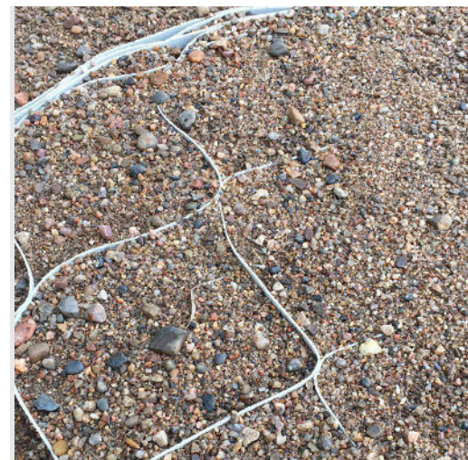
Tough Cell® infilled with 25mm gravel fill
