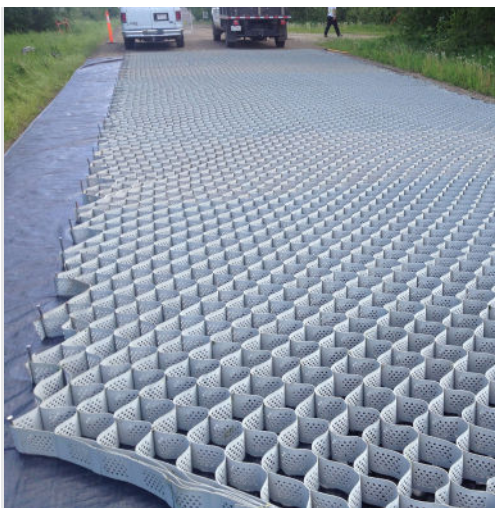
Typical placement of geotextile and Tough Cell® geocells
