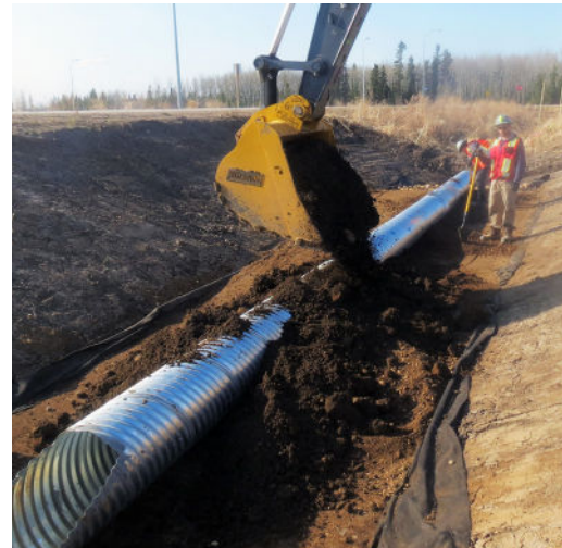
Preparation of drainage ditches.
