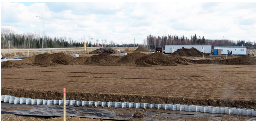
Yard area infilled and surfaced with gravel.
