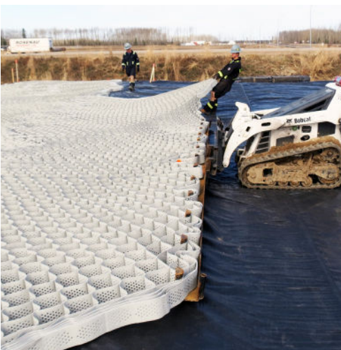
Installation of ToughCell ® over geotextile.
