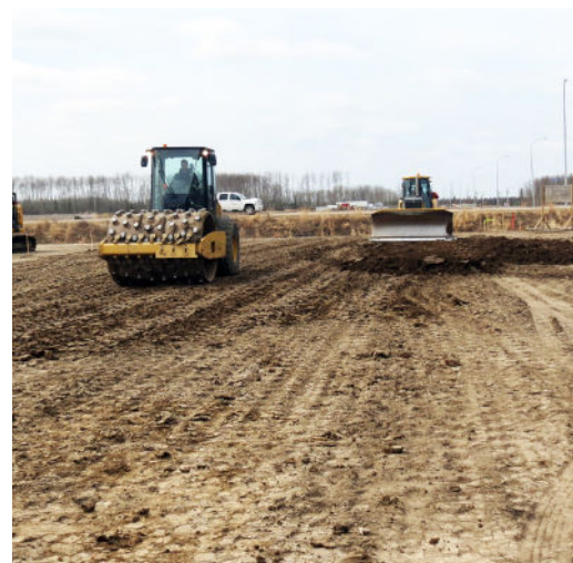
Infilling in progress.
