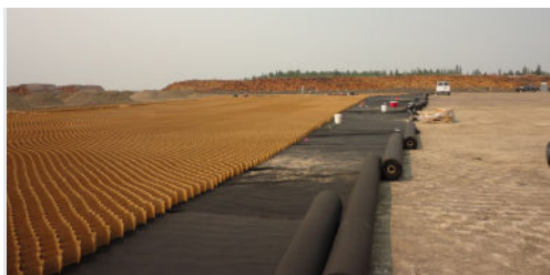
(top) Phase 3 site preparation
