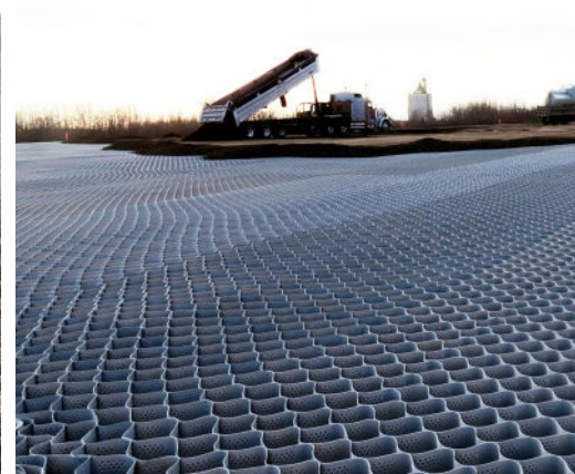
Phase 2 yard , Tough Cell® installed and being infilled
