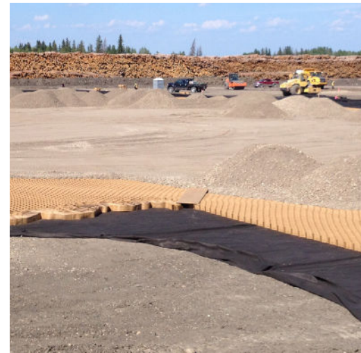
Completing Phase 3 infill
