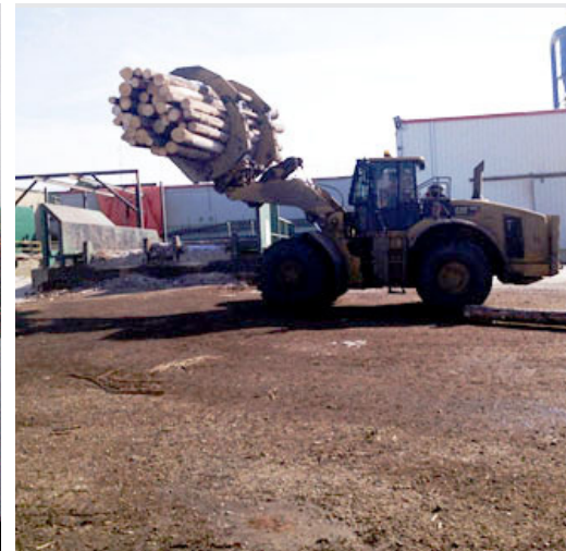
CAT 988 loader on completed Phase 1 surface
