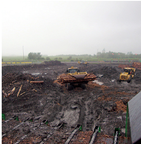
CAT 988 loader approaching hot deck prior to construction (Phase 1)
