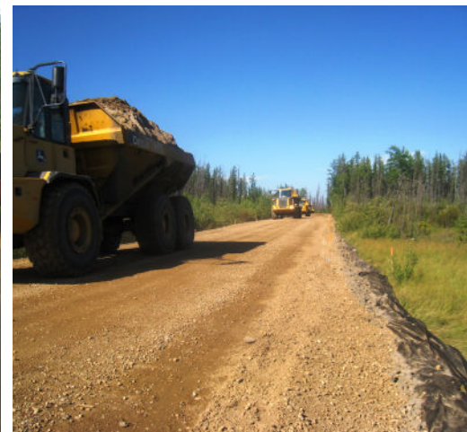
Completed road accepting heavy truck loads
