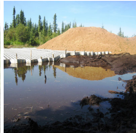
First layer Tough Cell® installed, ready for sand infill
