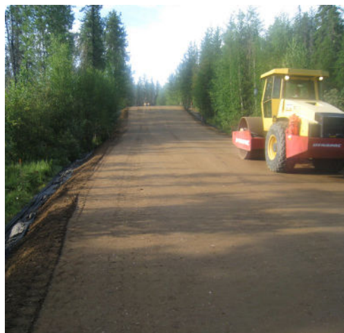
Final compaction of finished road surface
