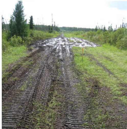
Condition of access route through muskeg
