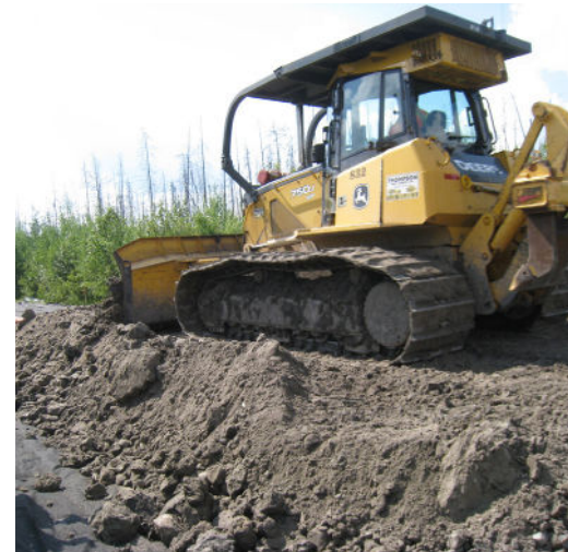
Second layer Tough Cell® infilled with gravel
