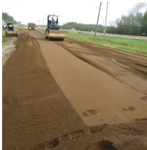
Compaction of sand base
