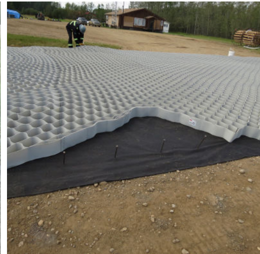
Installation of geotextile and Tough Cell®
