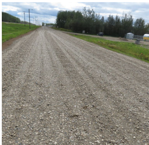
Completed road, August 2013
