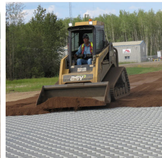
Infilling of Tough Cell® with track loader
