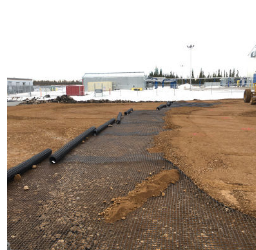
Installation, fill and compaction of geogrid layer
