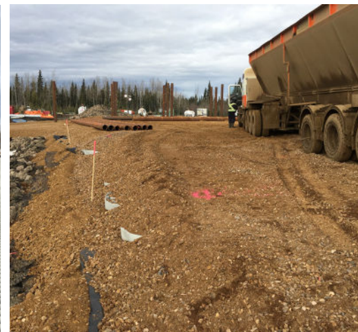
Gravel course and compaction
