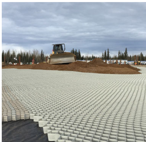
Infilling of Tough Cell® Geocells
