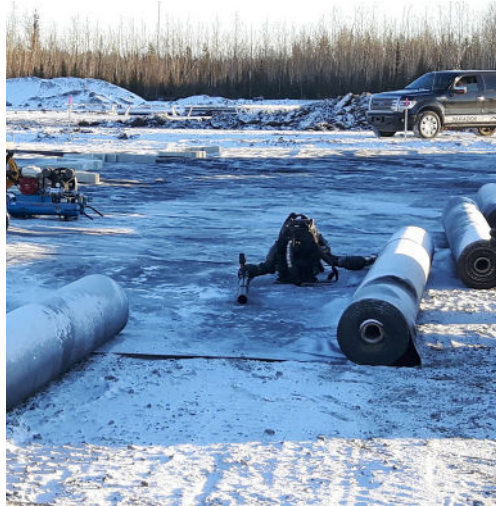
Installing geotextile in winter conditions
